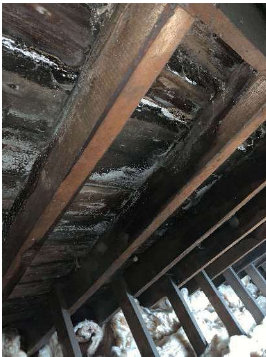
View from attic space showing rotten timbers
