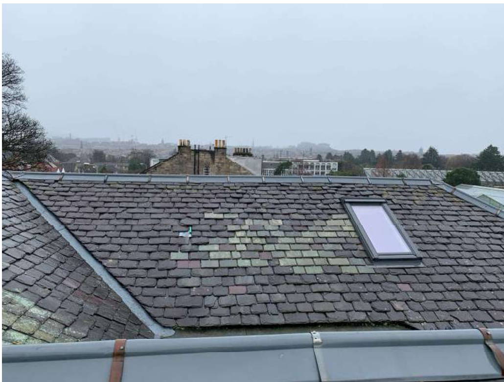
View from roof showing degradation of roof fabric including poor quality of localised repairs with alien roof tiles.
